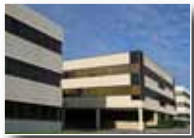
SECURITY OFFICE PARK Baltimore, MD
